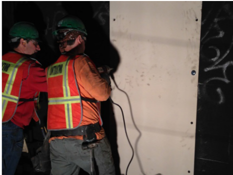
Figure 3 | Advantic+35 Panel Installation
